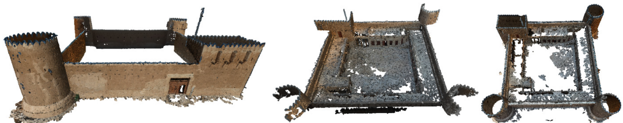
Figure 8: 3D point cloud of the exterior walls (left) and of the court yard (centre) from Bundler/PMVS2, and the entire point cloud of Al Zubarah fortress from VisualSFM (right)
