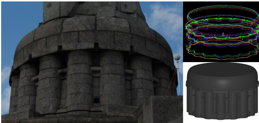
Fig. 5. Part of the socket of the Bismarck statue (left), generated cross-sections of the geometric object (right top), CAD model of the socket (right bottom)
